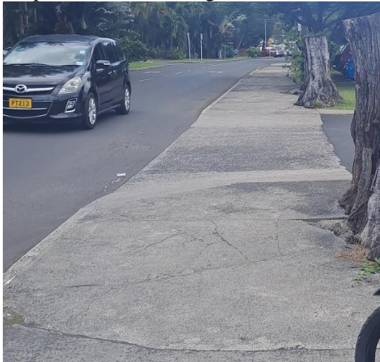
CITC Shopping Centre vehicle crossing (sloped)
