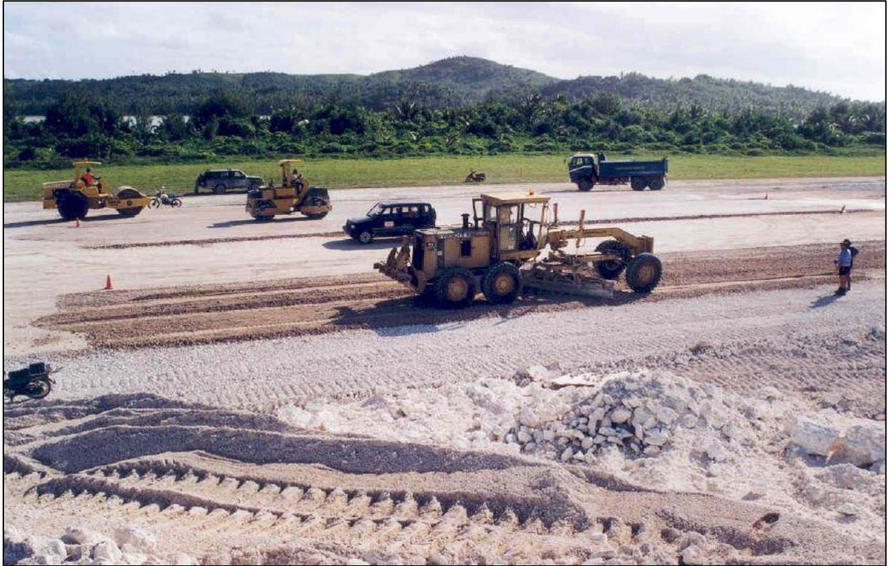
Figure 15: Grading the Aitutaki Runway 2004 (Source AACI)
