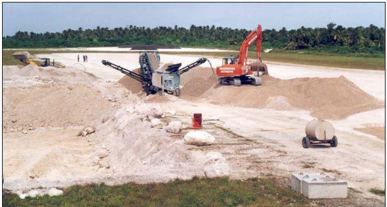
Figure 14: Quarry operations along the Aitutaki Runway 2004 (source AACI)
