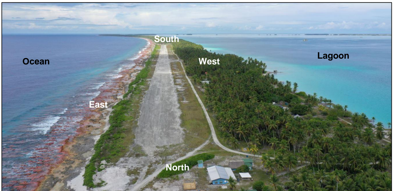
Figure 17: Aerial view of Manihiki Airport 2022 (source ICI PPP division)
