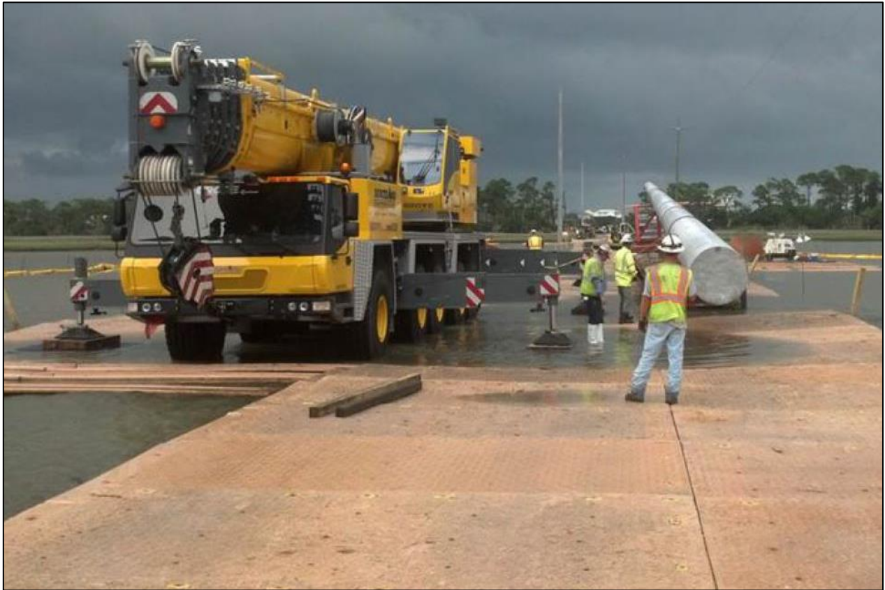
Figure 7: DURA-MATS used in USA around 2013 to access across tidal lakes.
