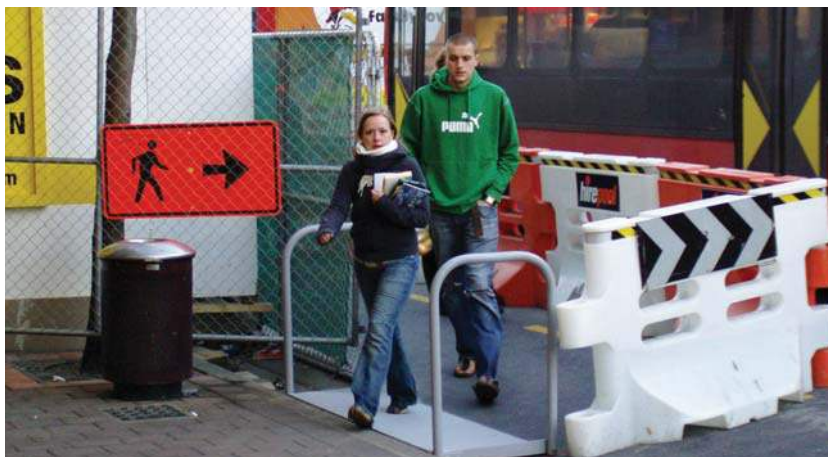
Photo 18.6 – Footpath diverted onto protected roadway with temporary kerb crossing and rail (Photo: Tim Hughes)
