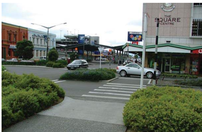
Photo 6.31 – Roundabout with zebra crossings on the approaches, Palmerston North CBD (Photo: Shane Turner)
