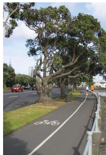
Photo 6.9 – Segregated path, Auckland (but substandard width)
