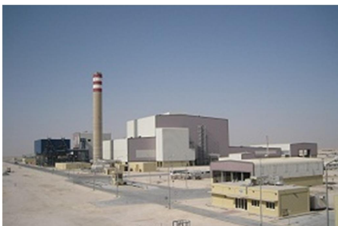
Exterior of a MSW Incinerator in Qatar
